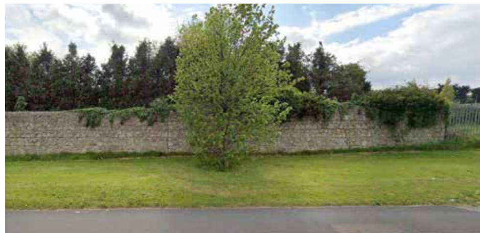
EXISTING RUBBLE WALL ALONG N11
